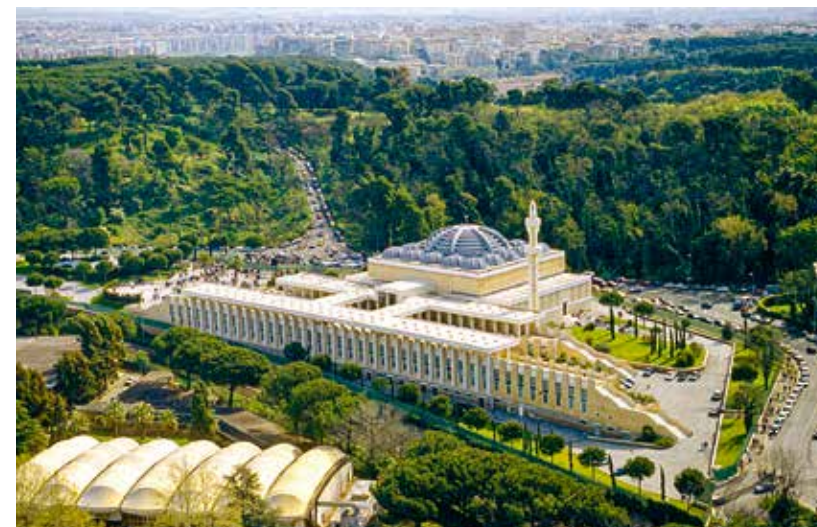
Figure 5. The Islamic Center and Mosque, Rome, Italy (1994)
