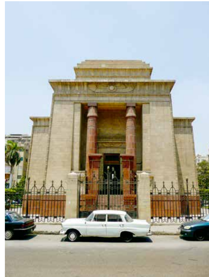
Figure 3. Sa'd Zaghlul Mausoleum, Cairo (1929): View from the east
