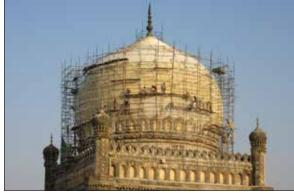
Conservation works on Sultan Quli Qutb Shah's Tomb (top) required replacing cement plaster with traditional lime plaster; and re-building of its garden enclosure wall after its original foundations were excavated (centre); Over 60 masons worked tirelessly to apply a traditional lime plaster layer on the dome of Muhammad Quli Qutb Shah (bottom).
