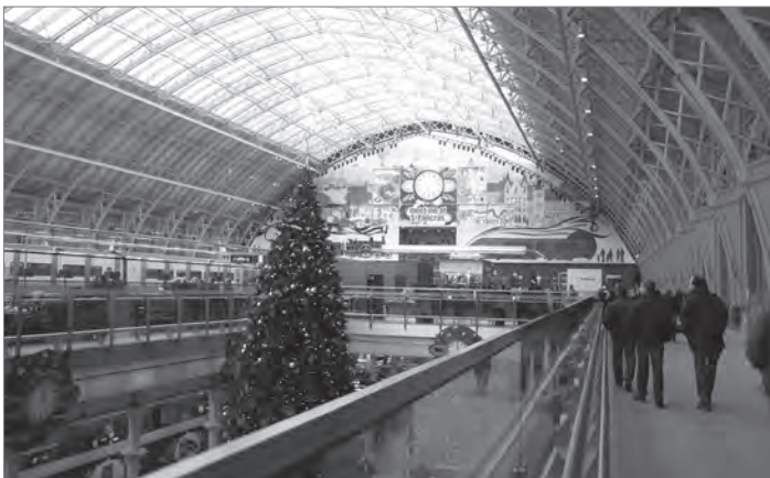
Fig. 1a: London, St. Pancras Station, William Henry Barlow, 1868; train shed.
