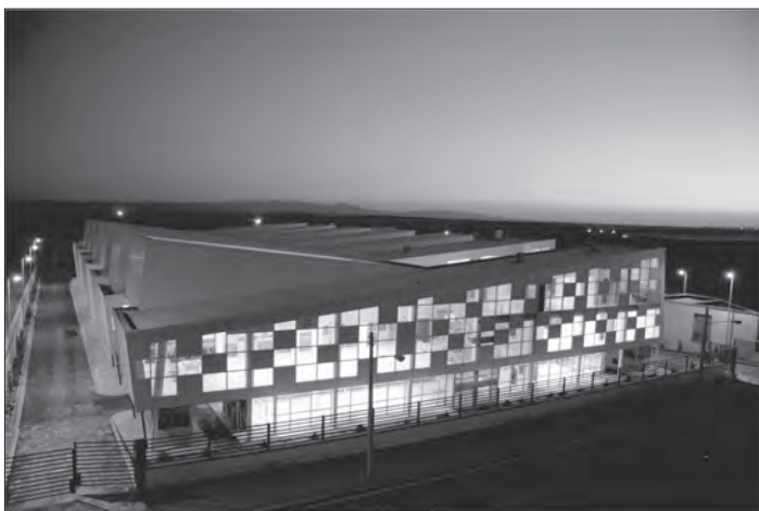
Fig. 42: Parand Industrial City, Peykar Bonyan Wood Paneling Factory, Bahram Kalantari and Kouros Dabagh, 2007.
