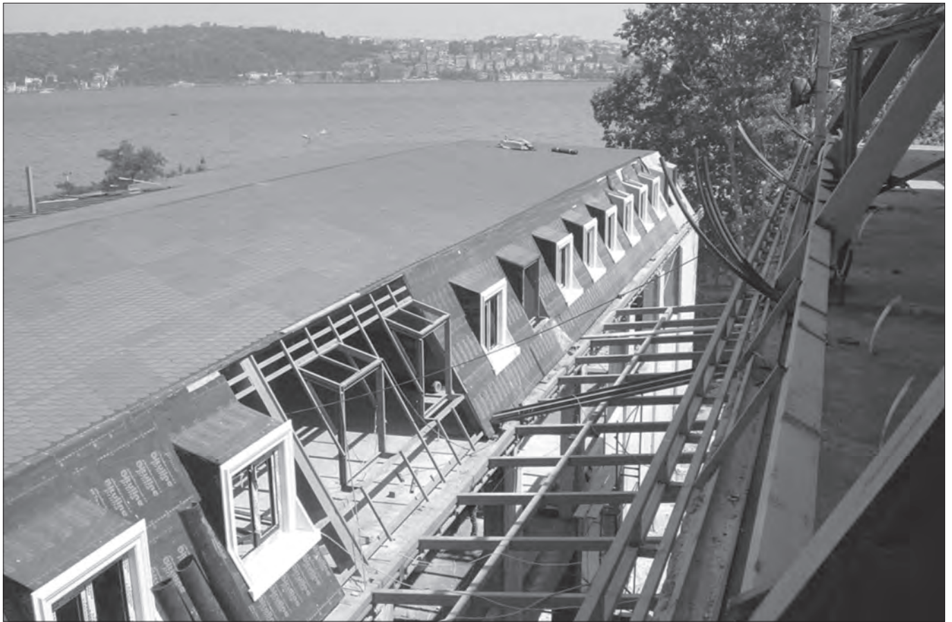
Fig. 22: BU Campus, view of the new roof under construction.
