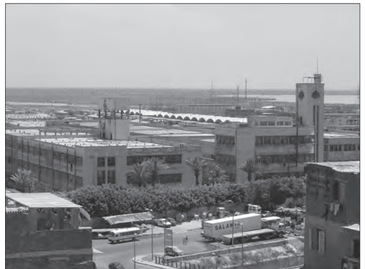
Fig. 52: Filature Nationale d'Égypte, new works, view from the north.
