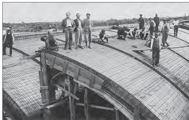
Fig. 25: Nazilli Cotton Textiles Plant, construction of the roof "fins," 1932–1936.
