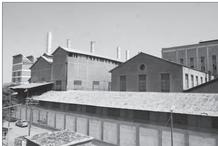
Fig. 21: al-Hawamdiyya, Sugar Refinery, originally founded in 1881; view of the northeastern section showing buildings dating from the early to the later 20 th century.
