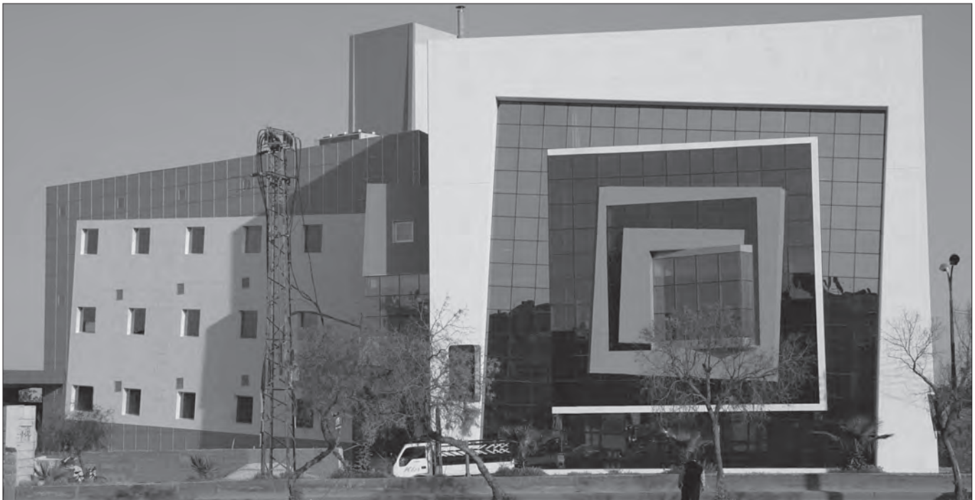
Fig. 19: The JG BLDG, street-front (north) view with the general manager's office projecting from the center of the concentric enframements.
