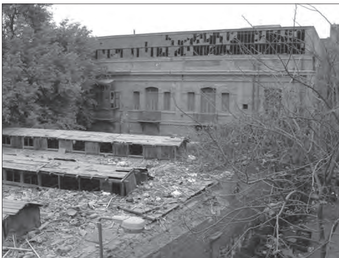
Fig. 35: Railway Telegraph Stores, view of northern facade.
