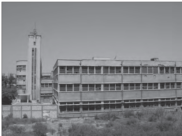
Fig. 53: Filature Nationale d'Égypte, new works, western factory block and office building with elevator tower.
