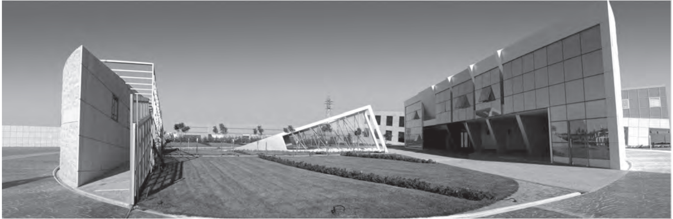
Fig. 11: The Chocolate Factory, view of the circular central court with its garden pavilion and the two segmental buildings to its right and left.
