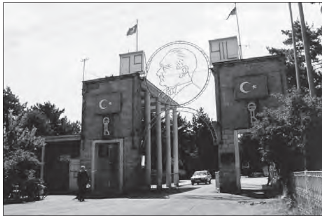
Fig. 18: Sümerbank Cotton Textiles Plant, monumental entrance.
