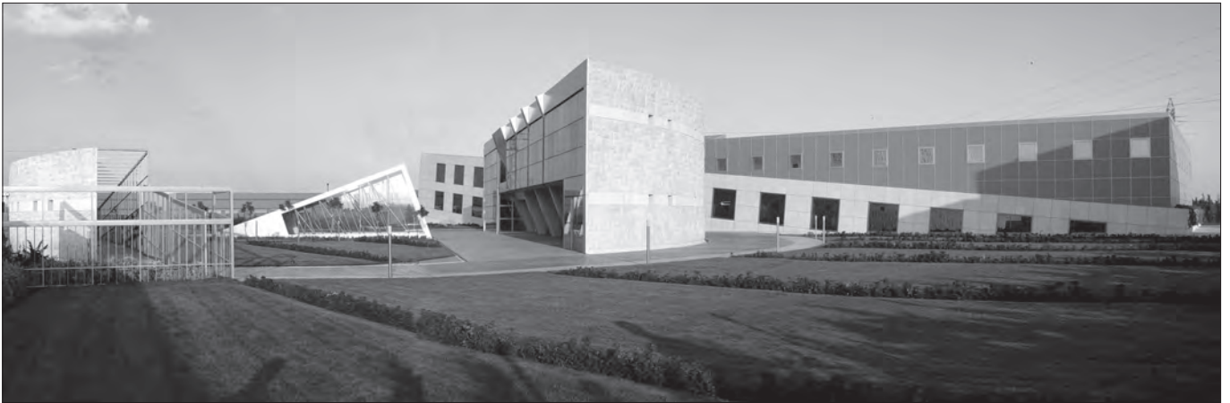
Fig. 8: The Chocolate Factory, panoramic view from the west showing the lush landscape and the dynamic profiles of the project components converging, diverging, and fanning out in different directions.
