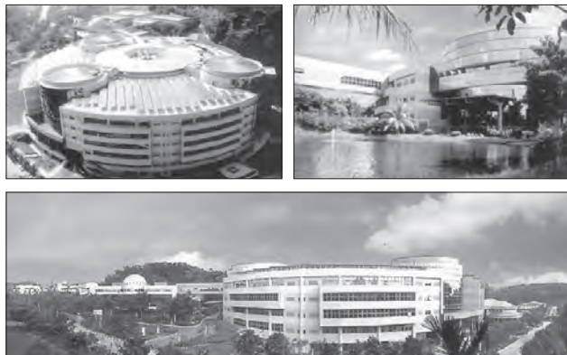
Fig. 11: Bukit Jalil, Technology Park Malaysia, Malaysian Institute of Microelectronics and Semiconductors (MIMOS), Ruslan Khalid Associates, 1997.
