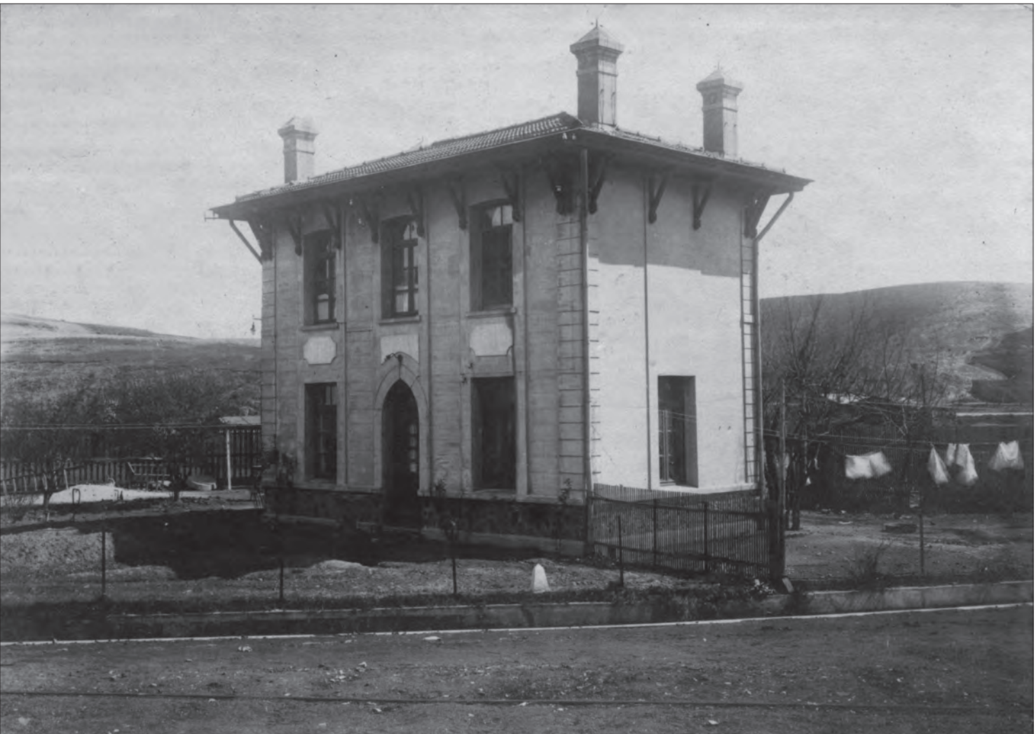
Fig. 9: Silahtarağa Power Plant, view of a housing building in the site.
