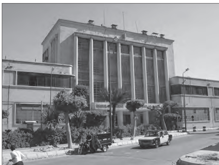
Fig. 59: STIA works, view of the northern block showing the administration building flanked by factory halls; the second floor of the factory halls was added in the mid-1950s.
