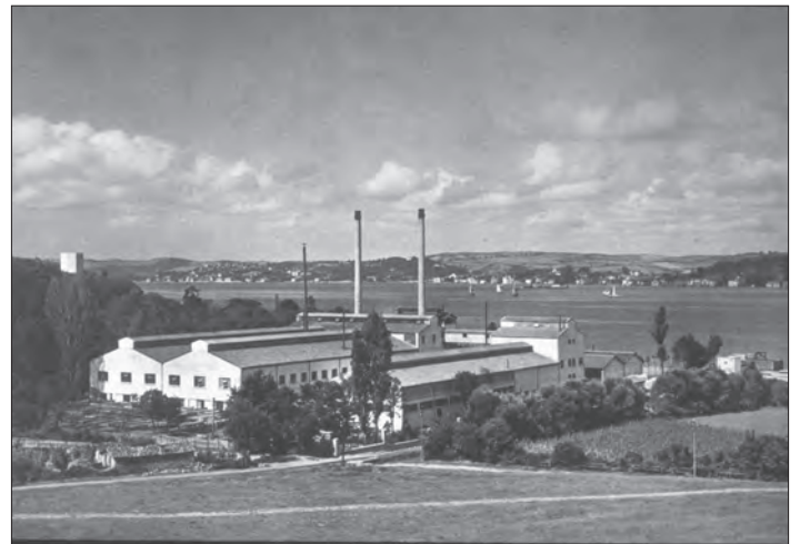
Fig. 2: İstanbul, Paşabahçe Glass Factory, 1934-1935.
