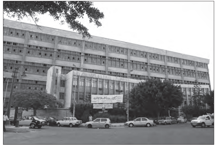
Fig. 69: Alexandria, Hadra District, STIA, new wool factory, Abu al-Fadl, Hadari, and Khuli 1974; view of the southern facades of the administration building and the central factory block facing Midan Sirri Pasha.
