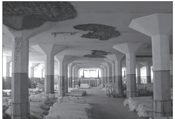
Fig. 61: STIA works, wool factory, Ferdinand Debbané, mid-1950s; interior view showing mushroom columns.
