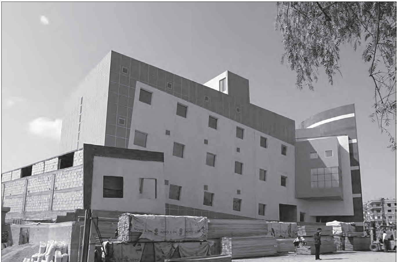
Fig. 21: The JG BLDG, general view from the east.
