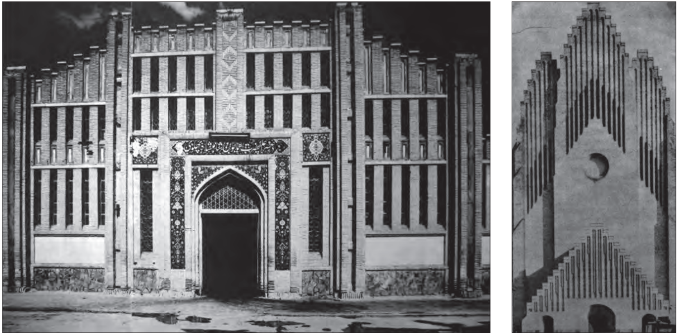
Fig. 7: Pair of images comparing the main entrance of the Risbaf Spinning Factory in Isfahan, c. 1935, to Grundtvig Church in Copenhagen, by Peter Wilhelm Jensen Klint, 1921–1940.
