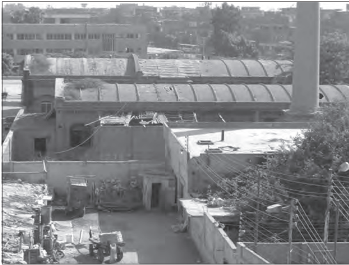
Fig. 42: Tanta Waterworks, ice factory, overhead view of the cylindrical "shell" roofs.
