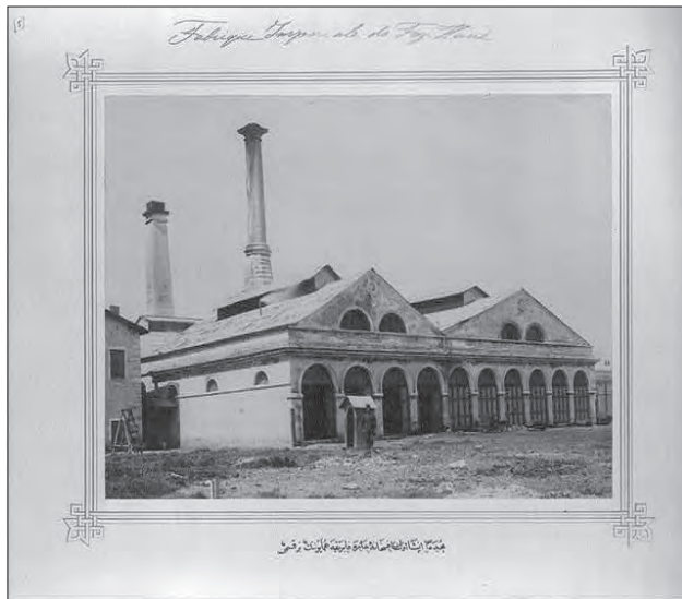
Fig. 4: Feshane, exterior of the boiler rooms.
