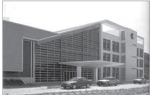
Fig. 9: Cyberjaya, Sepang, Selangor, George Kent Technology Centre, GDP Architects, late 1990s.
