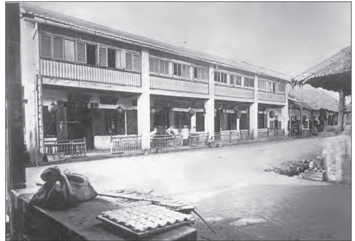
Fig. 3: The first shop houses in Market Square, Kuala Lumpur, c. 1884, were constructed using brick walls and concrete roof tiles by a Chinese 'Kapitan' (head of Chinese community), Yap Ah Loy.
