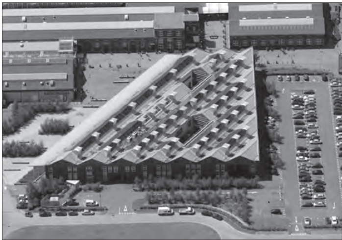
Fig. 11a: Swindon, National Trust Headquarters – Heelis Building, Feilden Clegg Bradley (structural engineers: Adams Kara Taylor), 2005.
