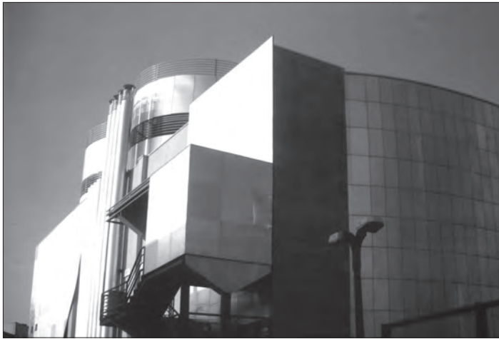
Fig. 40: Shiraz, Gas Company Headquarters, Mehrdad Iravanian, 2001.
