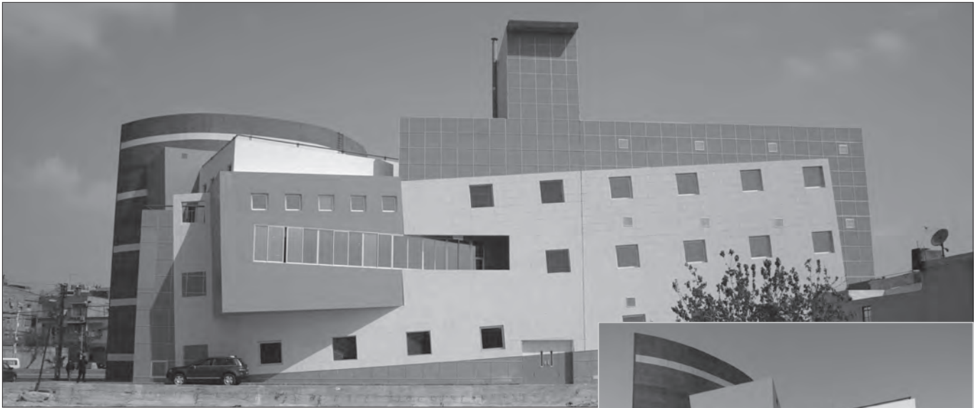
Fig. 22: The JG BLDG, view from the south showing the interlocking articulation and interconnection between the storage section to the right and the offices to the left.
