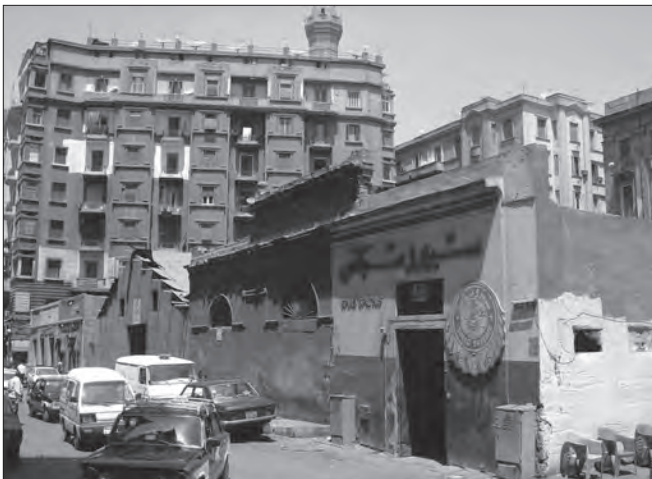
Fig. 38: Cairo, Bab al-Hadid District, Spiro Spathis Soft-Drinks Factory, first decade of the 20 th century; view of street facade.
