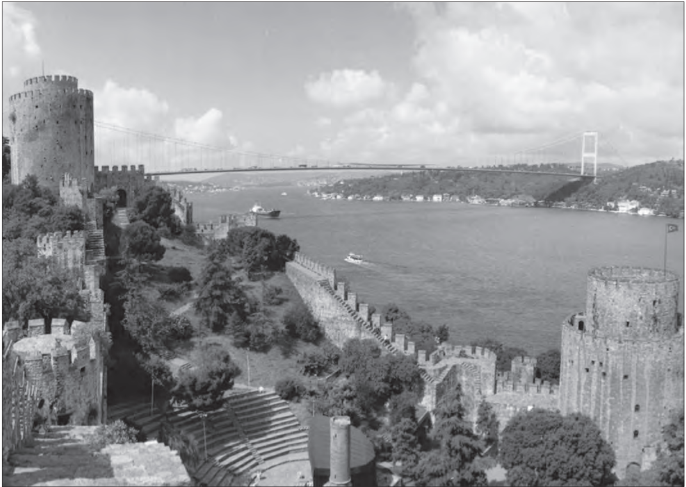
Fig. 3: İstanbul, Rumeli Hisari, an example of an Ottoman seashore military structure in the city.
