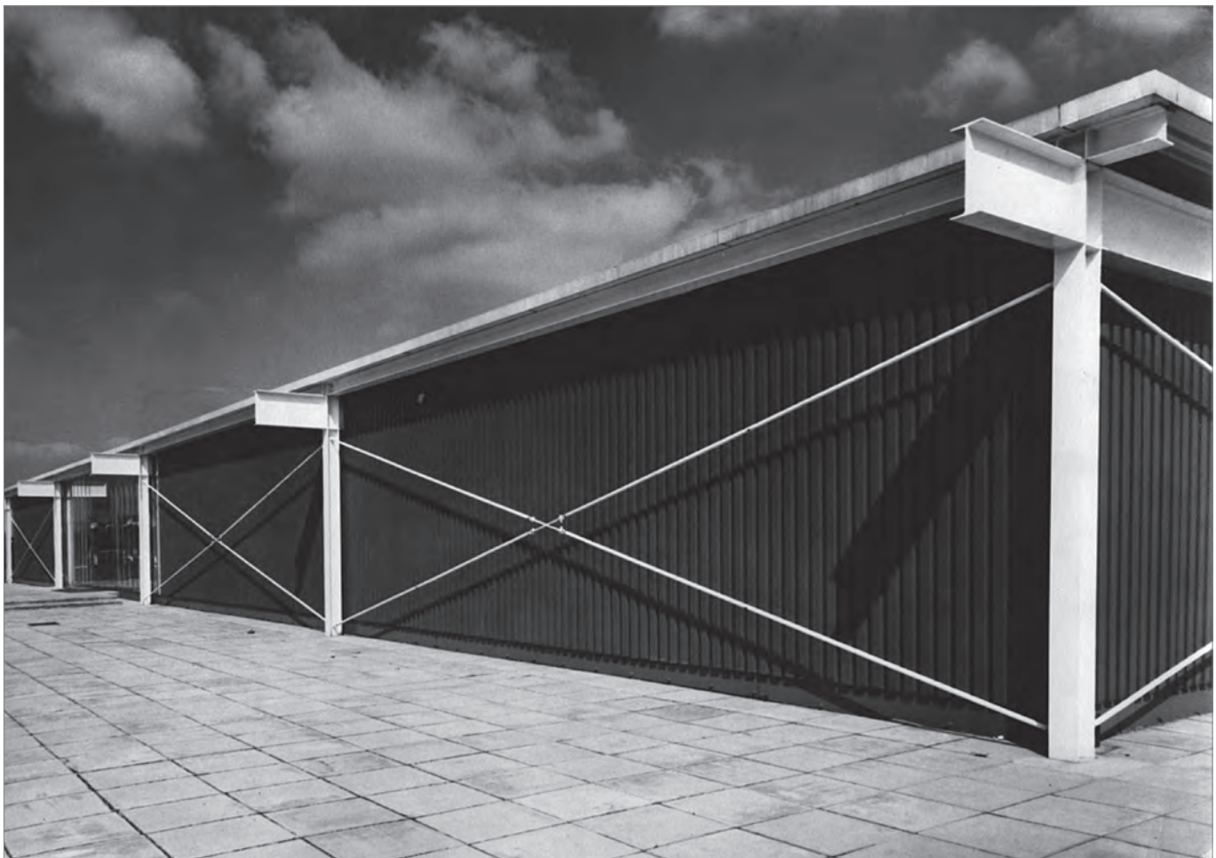
Fig. 2: Swindon, United Kingdom, Reliance Controls Factory, Team 4, 1967.
