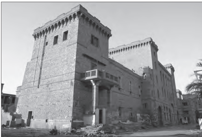
Fig. 32: S. A. Brasserie des Pyramides Brewery, view of western annex and central block.
