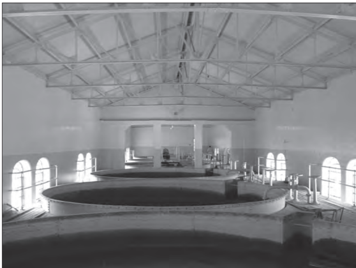
Fig. 43: Tanta Waterworks, interior of the filter and pump house.
