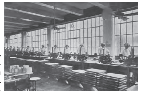
Fig. 2b: Ford Motor Company Engineering Shops, the windows of the Engineering Shops provide natural light and ventilation.
