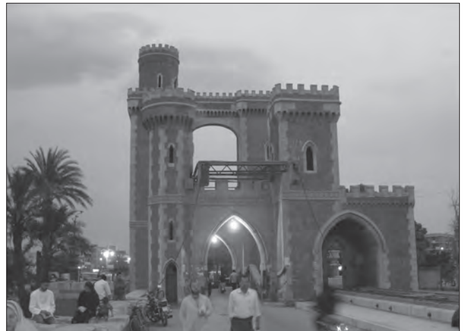
Fig. 26: al-Qanatir al-Khayriyya, eastern gate tower of the Delta Barrage, 1862.
