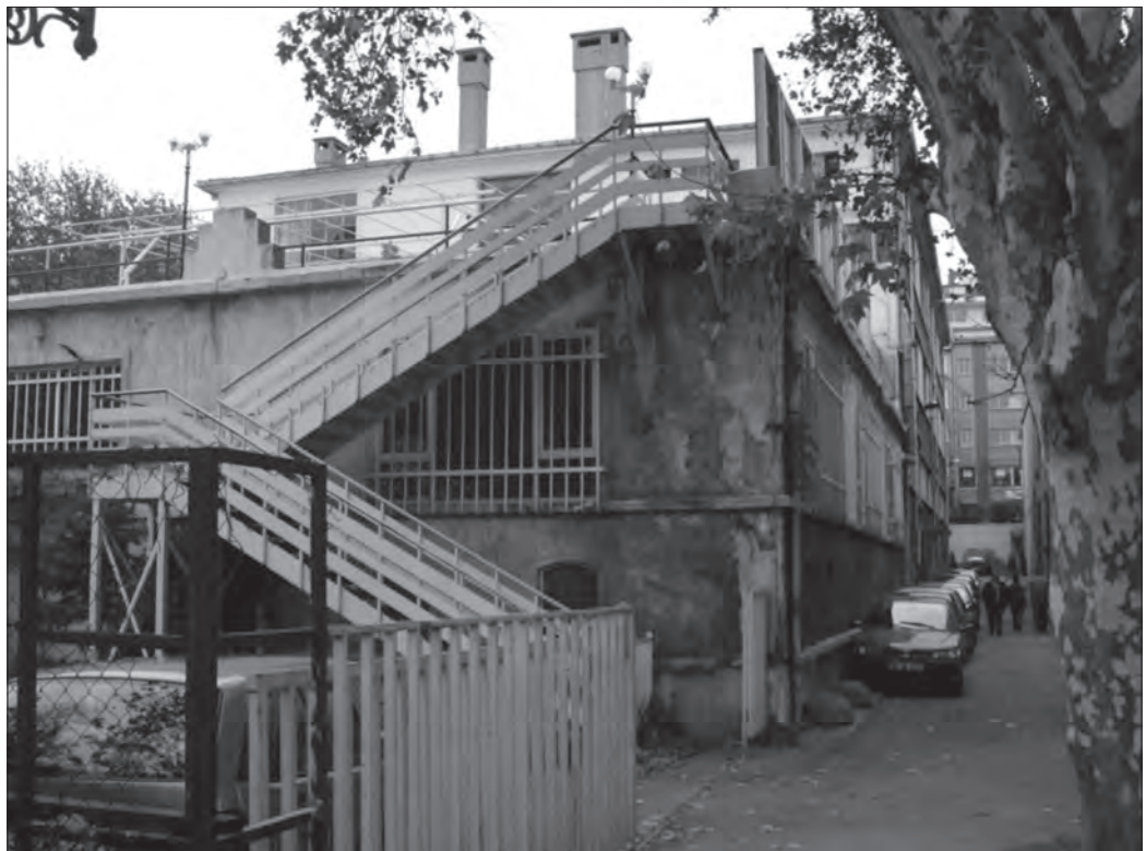
Fig. 11: BU Campus, view from the seashore side of the narrow street located between the two warehouse buildings prior to their conversion.
