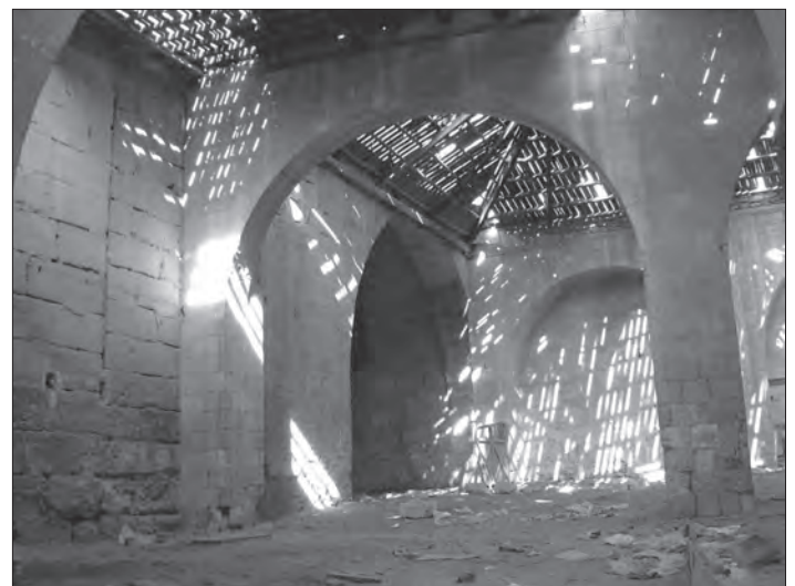
Fig. 5: Citadel Arsenal, gun foundry, workshop hall with stone arcades.
