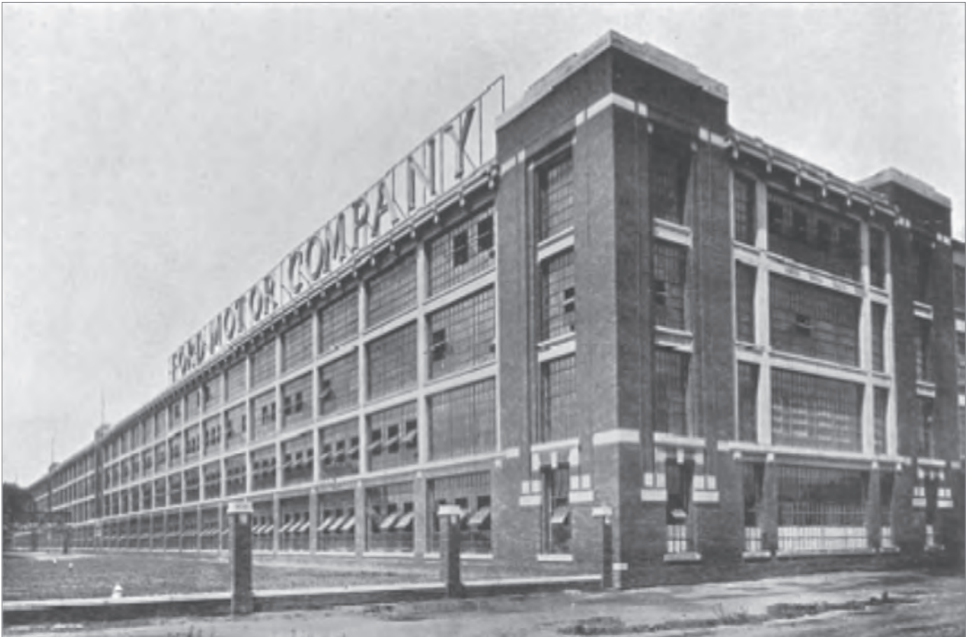
Fig. 2a: Dearborn, Michigan, Ford Motor Company Engineering Shops, Albert Kahn, 1917–1928; the external articulation of windows provides an example of an economically-produced architectural effect.
