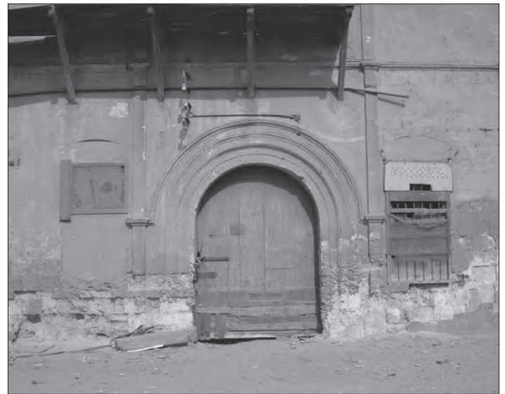
Fig. 4: Citadel Arsenal, gun foundry gate, 1820s.
