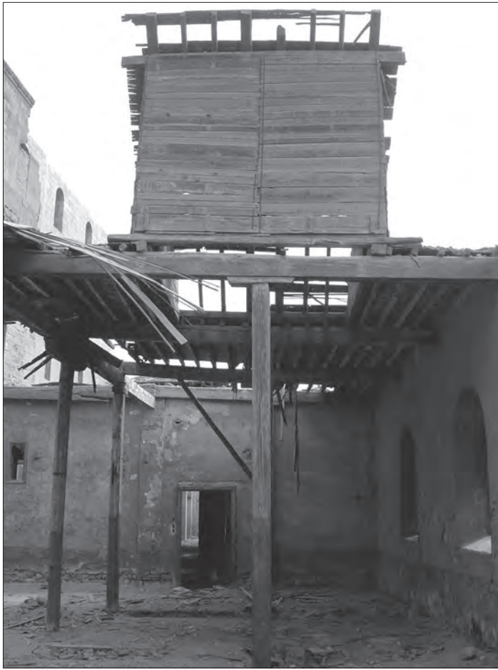
Fig. 6: Citadel Arsenal, workshop hall next to the gun foundry, view of timber roof with malqaf .
