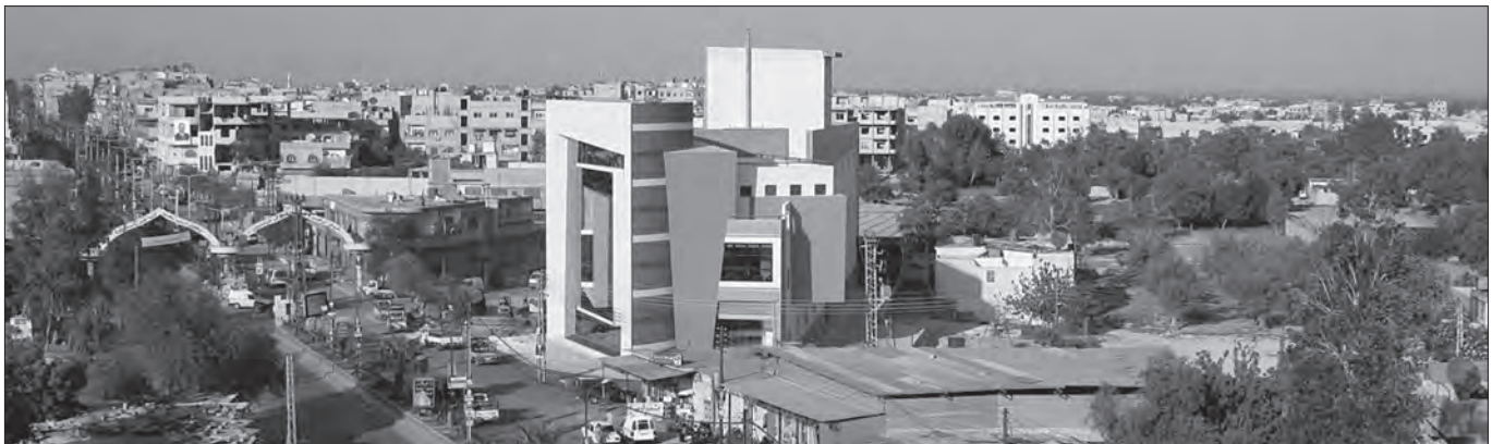
Fig. 18: The JG BLDG, general view from the west.
