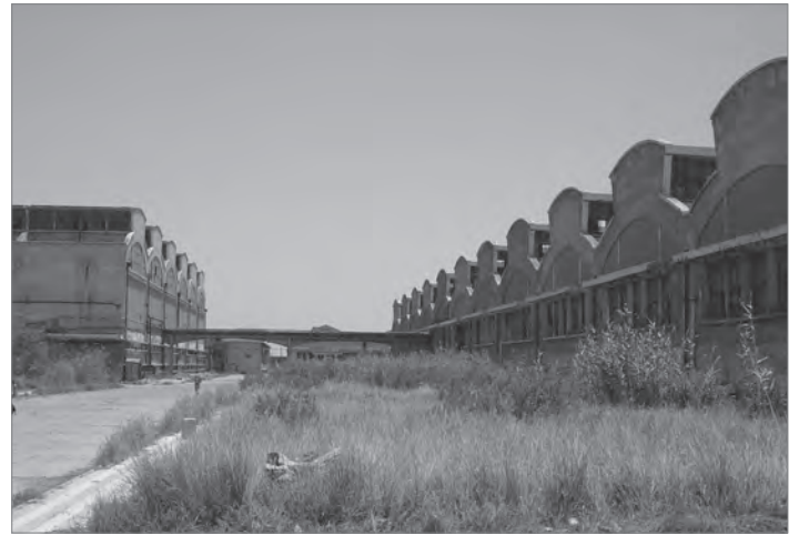
Fig. 63: al-Shirka al-Ahliyya, view of 1962 extensions, with new dye works for cloth (right) and for yarn (left).
