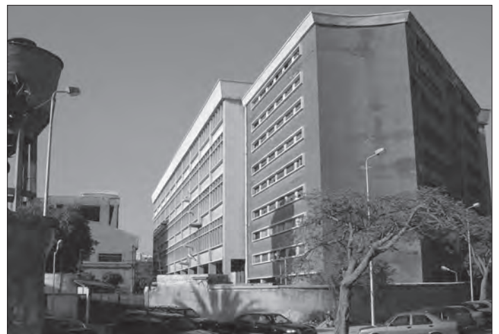
Fig. 70: STIA, new wool factory, view of the trapezoidal annex and central factory block from the west.
