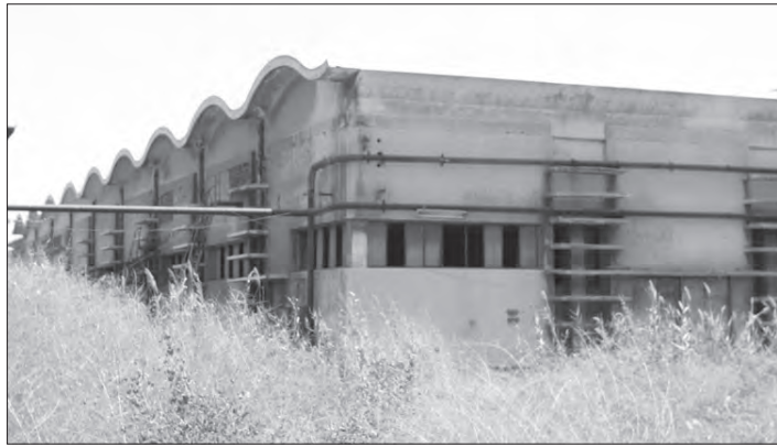
Fig. 68: al-Shirka al-Ahliyya, 1962 extensions; view of generator building with undulating multi-barrel shell roof.
