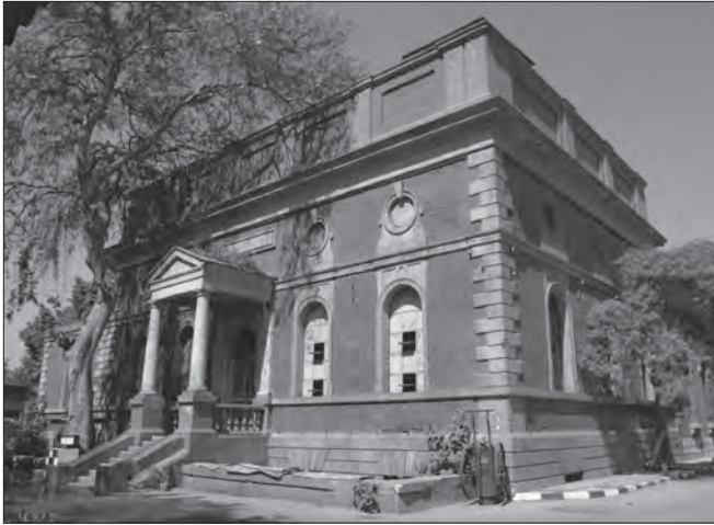
Fig. 36: Giza, Waterworks, pump house, 1896.
