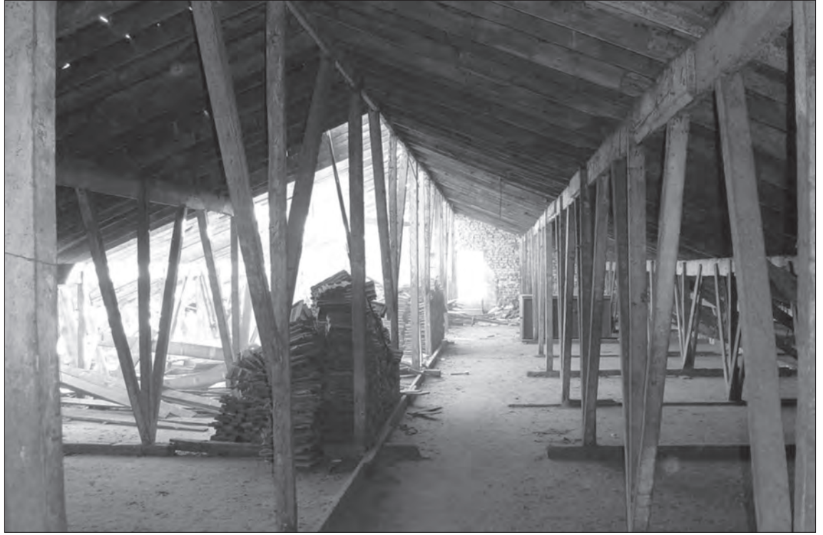
Fig. 21: BU Campus, view of the old roof.
