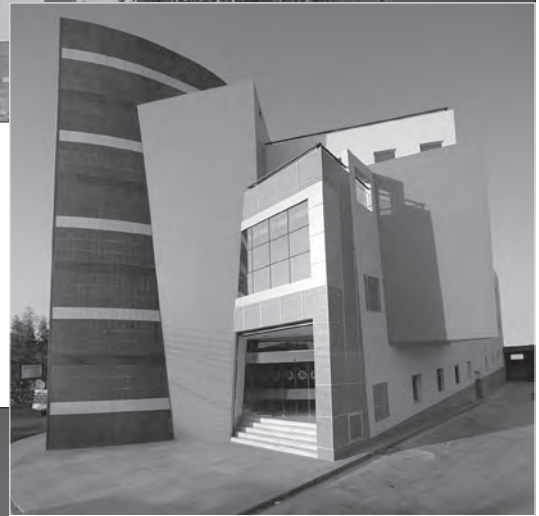
Fig. 23: The JG BLDG, detailed view from the west showing the main entrance.
