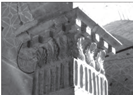
Fig. 27: Harati Textile Factory, column detail.
