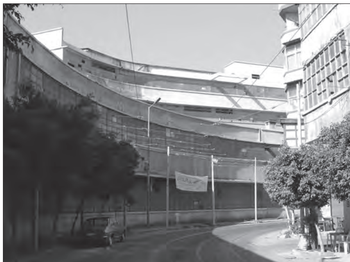
Fig. 58: STIA works, street façade view of the southern blocks.
