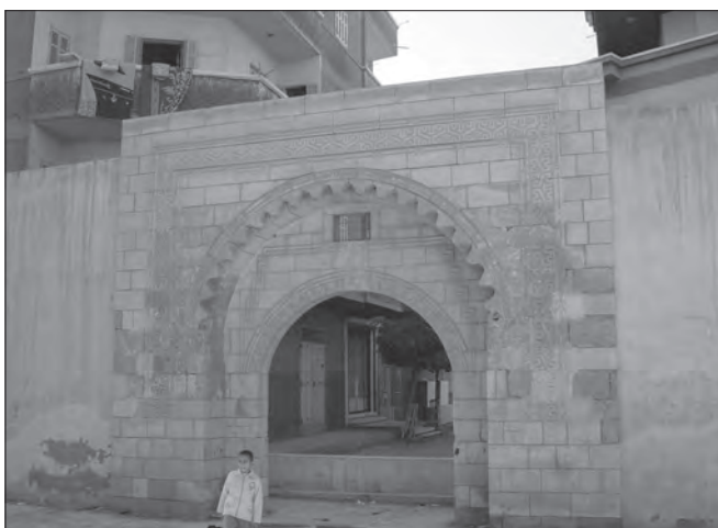
Fig. 14: Tarbush Factory, interior gate.
