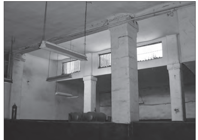
Fig. 39: Spiro Spathis Soft-Drinks Factory, interior view of the 1926 addition showing stone columns and monitor roof.
