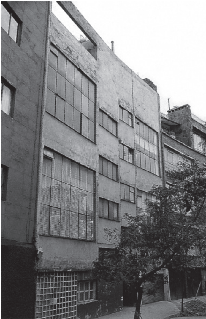
Figure 15: Barragan building from the 1930s.
