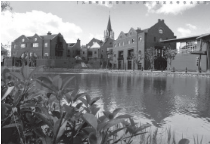
Figure 3: Views of Thames Town, Songjiang City, China.
