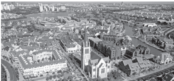
Figure 1: Aerial view of Thames Town, Songjiang City, China.
