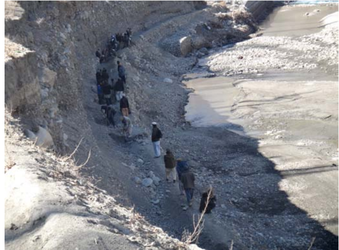
Communities participating in repairing water channels
