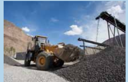
160,000 Cubic Metres of Rock Being Cleared at Khorog Campus Site
