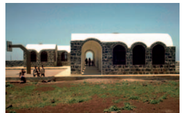
Stone Building System, Dar'a Province, Syria, 1992
