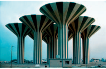
Water Towers, Kuwait City, Kuwait, 1980
