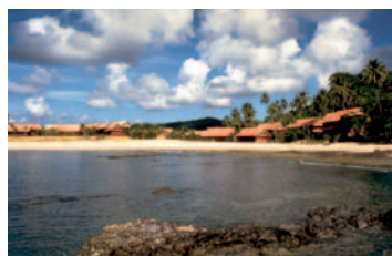
Tanjong Jara Beach Hotel and Rantau Abang Visitors' Centre, Kuala Terengganu, Malaysia, 1983
