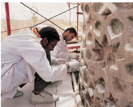
(Top) The mosque and minaret of Khayer Bek is part of a larger monumental complex under restoration by AKTC. (Above) Cleaning and restoration of the decorated shaft of the Khayer Bek minaret was a painstaking endeavour.
