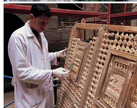
(Top) The minaret of the fourteenth-century Um al-Sultan Shaaban Mosque has recently been restored by AKTC, including reconstruction of its top pavilion. (Above) Restoration work in the Khayer Bek complex: a wood conservation workshop was set up on site to restore the numerous mashrabiyya screens found throughout the complex. (Below left) The ongoing cleaning and restoration of a decorated wooden ceiling.
