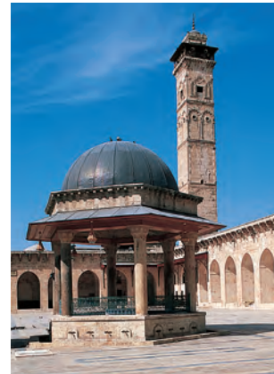
(Top) The Mosque as seen in an early twentieth-century photograph, before restoration. (Above) The Great Mosque of Aleppo as seen after recent restoration work.
