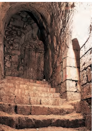
(Top) The remains of the entrance to the Ayyubid well (satura) (above) with a staircase going down 52 metres to the level of the moat and water table (right) as shown in the section.
