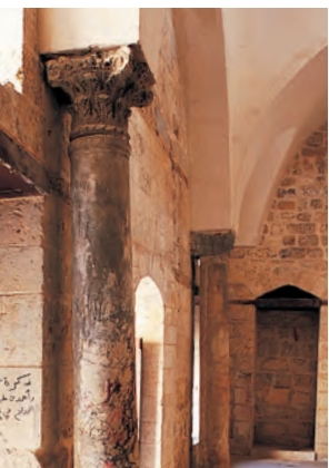
Reuse of a Byzantine column and capital in the prayer hall of the Mosque of Abraham.
