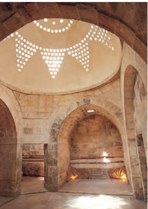
The interior steam room of the Palace Hammam. Several coats of plaster show ongoing maintenance during the mediaeval period.
