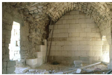
During 2000, conservation work focused on the flanking tower, a small vaulted space on the west wall (above left and middle). The inner layer of stonework had collapsed, and was entirely rebuilt. In 2002, HCSP will begin conservation work on the marble floor of the Ayyubid palace
