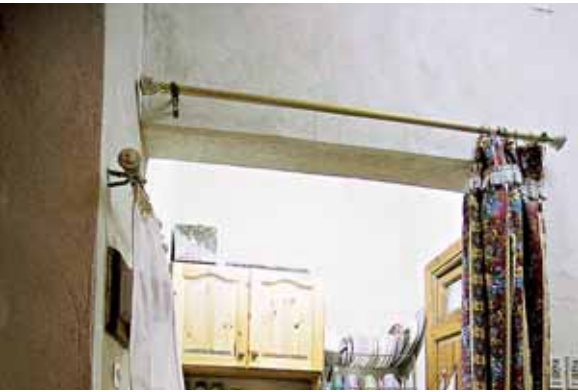
Apartment houses in Darb-al-Ahmar being renovated, and below, a refurbished kitchen in one of the upgraded houses.
