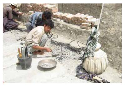
Restoration has involved the removal of reinforced concrete from the mosque roof.
