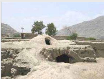
The ruined hammam prior to restoration
