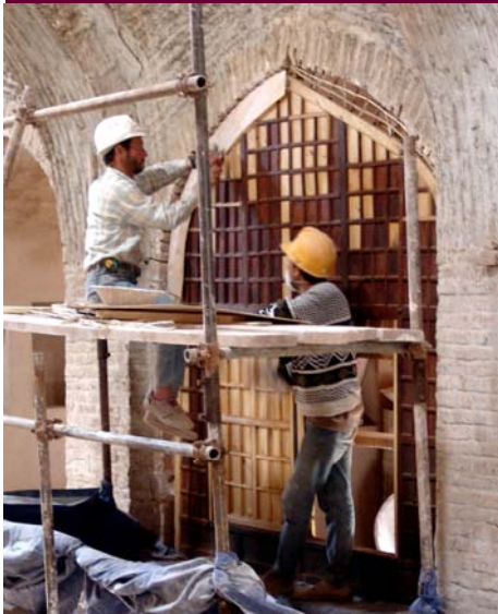
Restoration of damaged orosi screens on the first floor of the interior space has provided an opportunity to train carpenters
