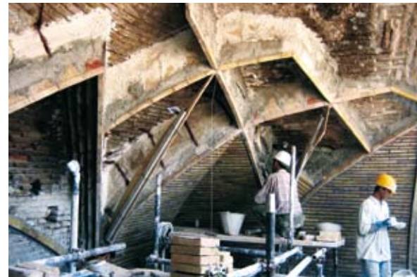
Inspecting repairs to the main dome over the Châhâr Suq Cistern and restoration work on the main entrance iwan of the complex.
