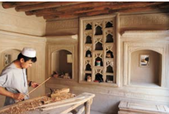
Carpenters at work repairing timber lattice-work screens.
