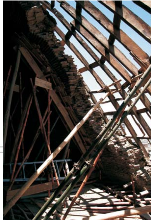
Prior to removal of unstable brick masonry, the damaged upper dome was propped.
