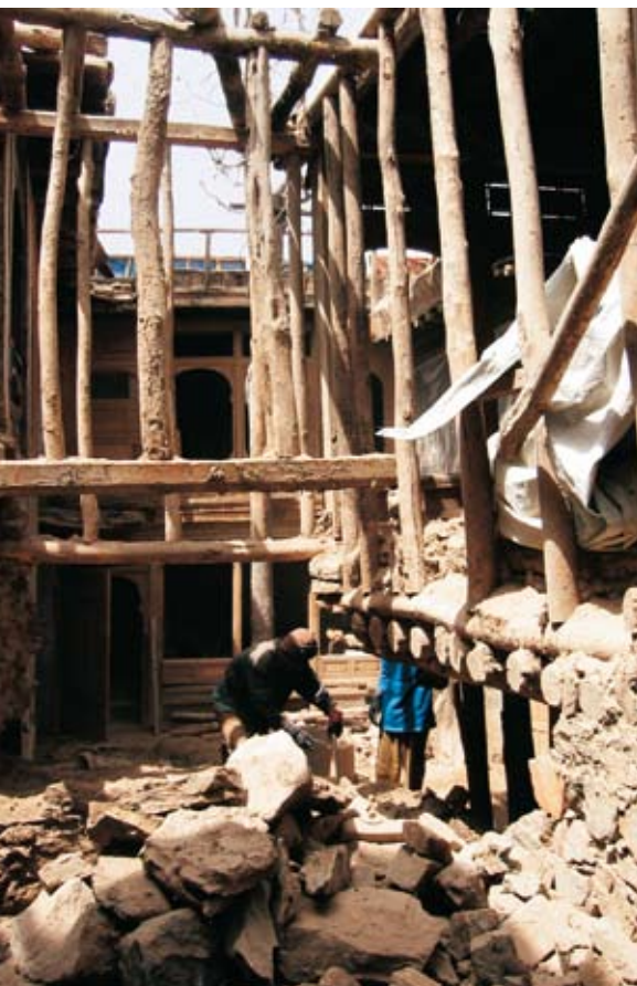
Brick infill is removed from the timber structural frame during restoration of the Shekiba house.
