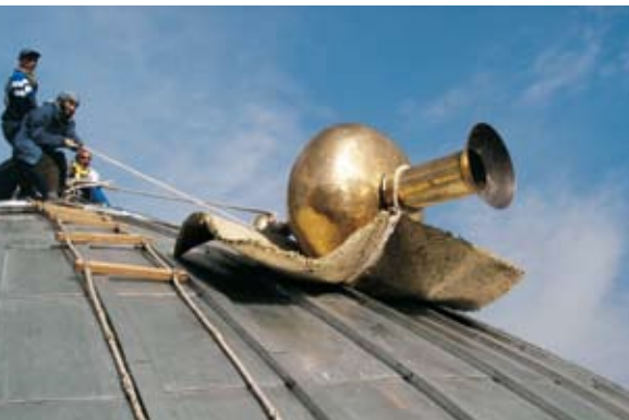
The repaired finial being raised to the apex of the dome and, below, the restored mausoleum with its new terrace at ground level.
