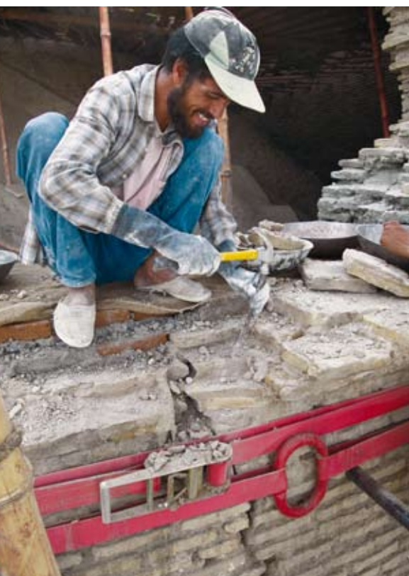
The drum of the upper dome was temporarily strapped during repairs to the masonry, for which specially fired bricks (below) were set in lime mortar.
