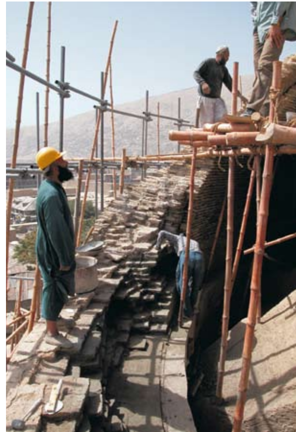
New brickwork being laid to match the coursing of the original dome.
