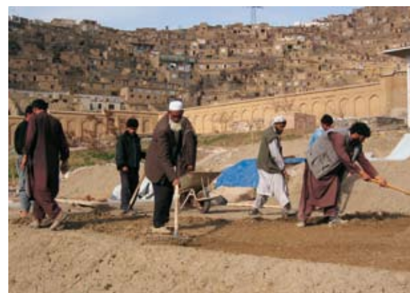
The northern verandah of the Queen's Palace nearing completion and, below, workers levelling the upper garden terraces prior to laying of turf.
