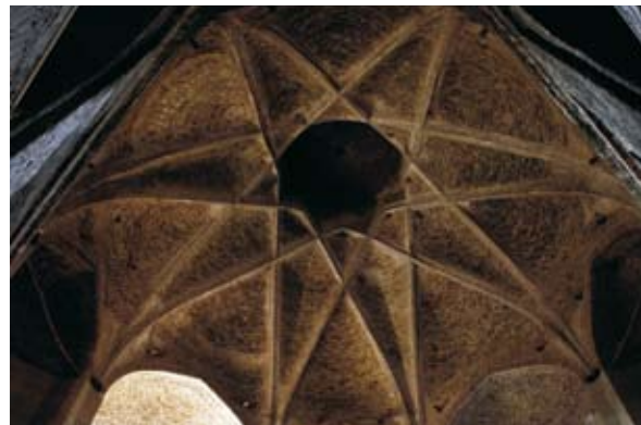
The ribbed brickwork on the inner side of the lower dome.
