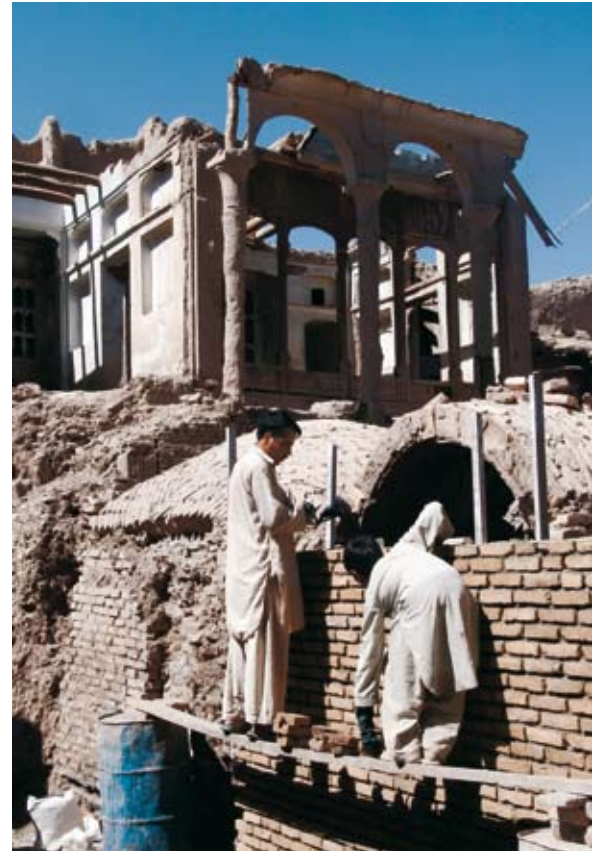
Reconstruction of brick vaults over the hammam wing of the Attarbashi house.
