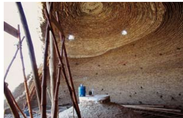
The interior of the upper dome shows signs of having been built in stages.
