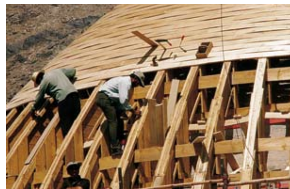
Fixing timber planking to the radial rafters, before galvanised iron sheeting was laid over the dome.
