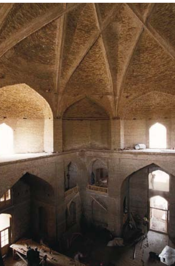
Interior of the mausoleum during restoration, showing the ribbed inner dome, built in brick.
