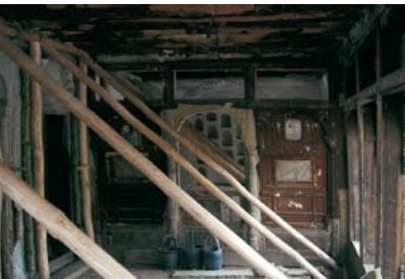
Deflection of the internal walls and timber screens (above) on the first floor of the Wasay house and props in place during stabilisation.
