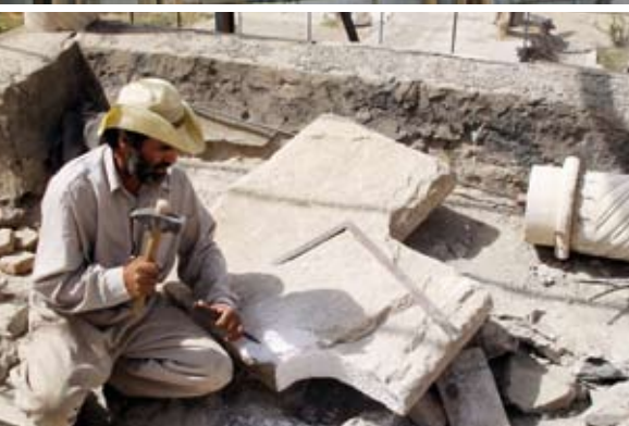
Left: A mason prepares a marble structural element as part of repairs to the war-damaged roof of the Shahjahan Mosque.
