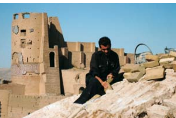
The Malik Cistern and Mosque complex under restoration and, below, preparing bricks for use on repair to the roof of the cistern.
