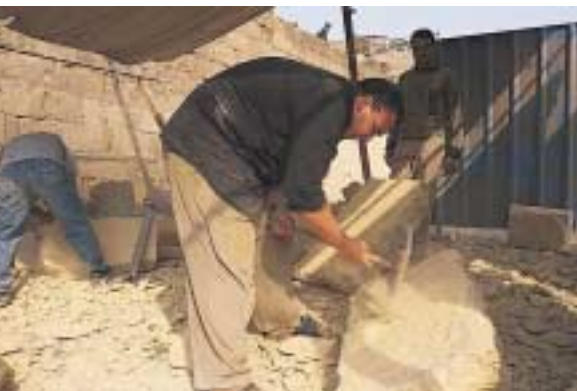
Above: Mason cutting stone for the wall restoration project.
