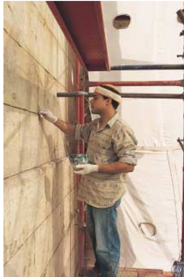
Replacement of cement by lime mortar in the joints of recent masonry.
