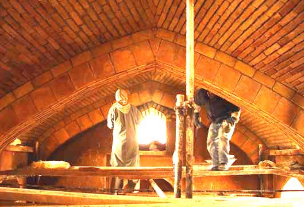
Masons finishing the brick arches and vaults in the main prayerspace
